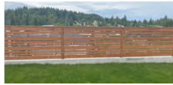
Dia. A - Typical perimeter and yard separation stained fence
